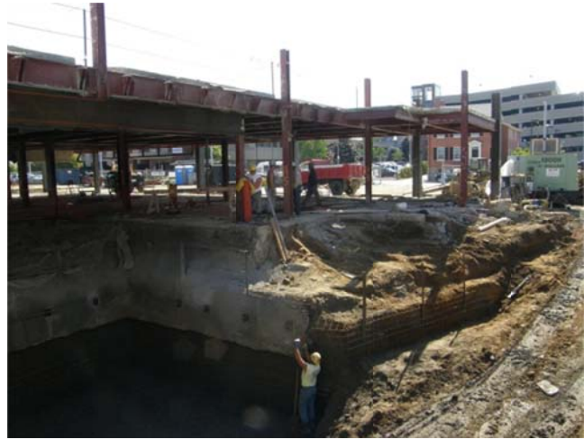
Figure 4: Foundation Excavation during Construction
